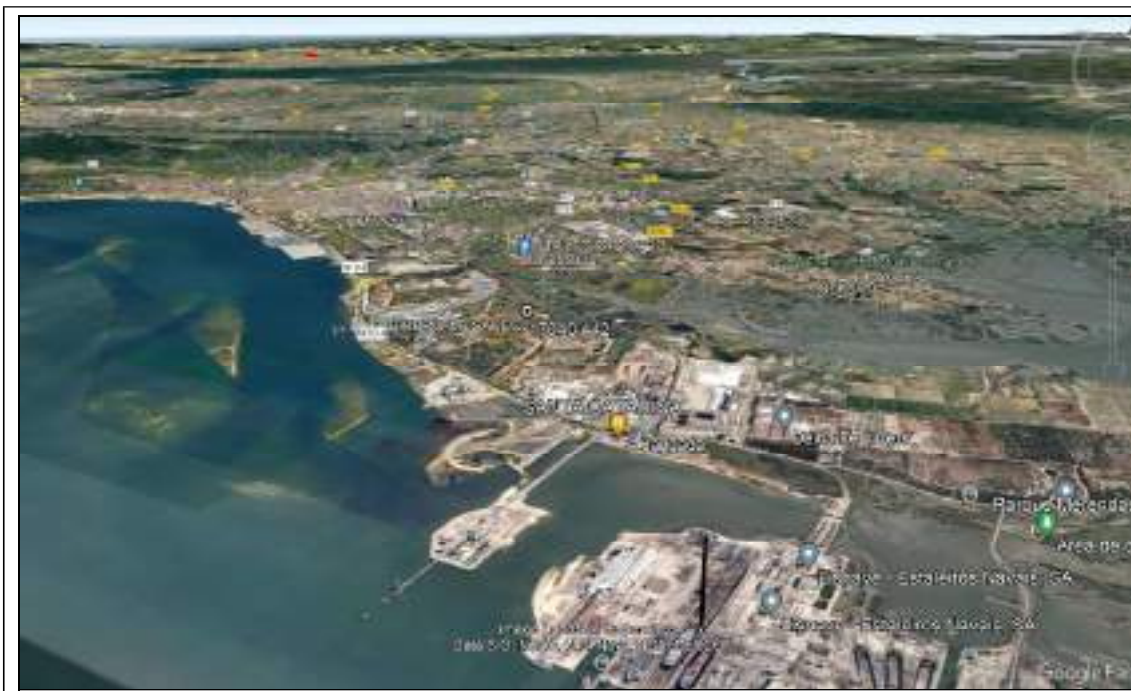
Figure 3 – Illustrative image of the geomorphology around the construction site.
