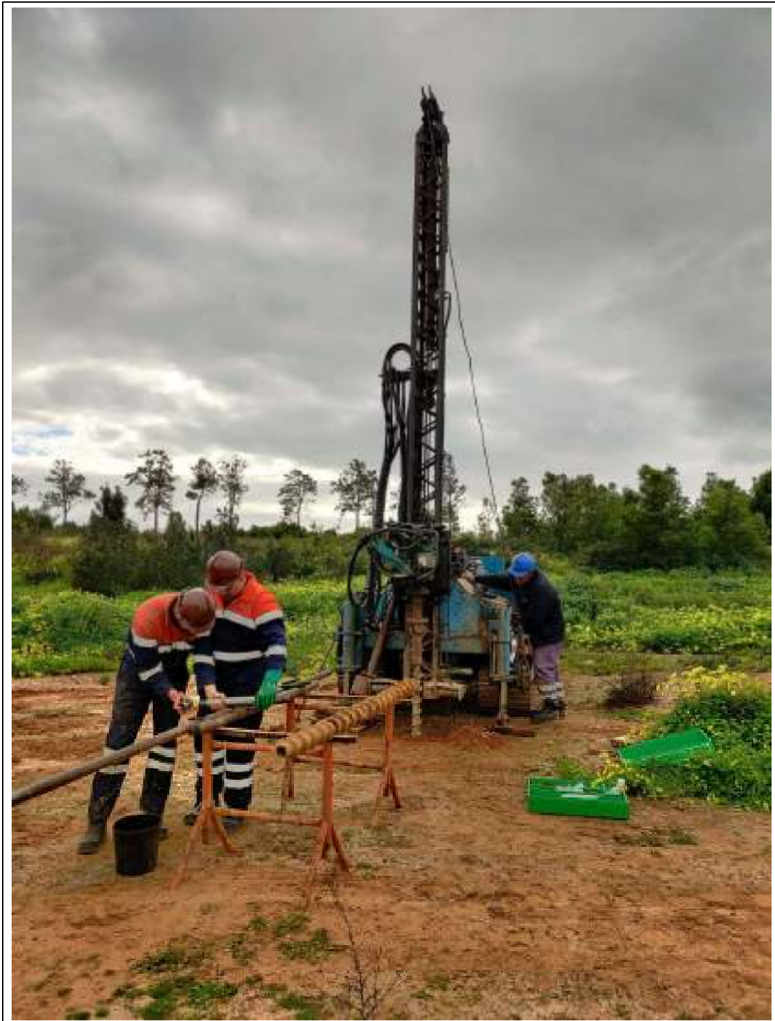
Figure 5 - Drilling equipment used (Edeco T-30)
