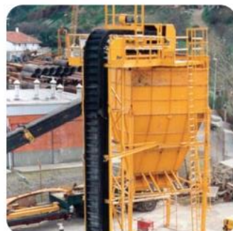
Civil work | Chile
