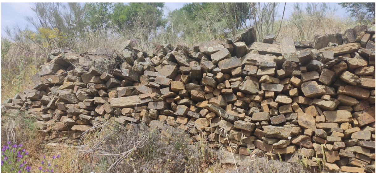
Figure 63: Terraced walls made of schist slabs on the southern slope.
