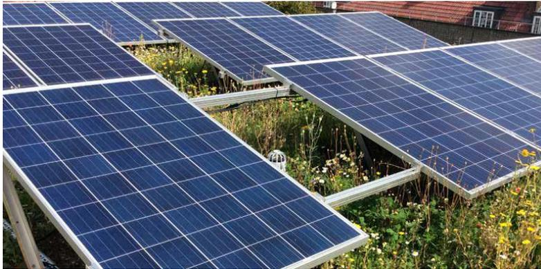
Fonte: BioSOLAR Integrated Green Roof Solar Panel System – Bauder
