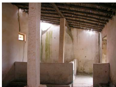
59 – Oc. 17, Fase 1 – CH, 1 no interior
