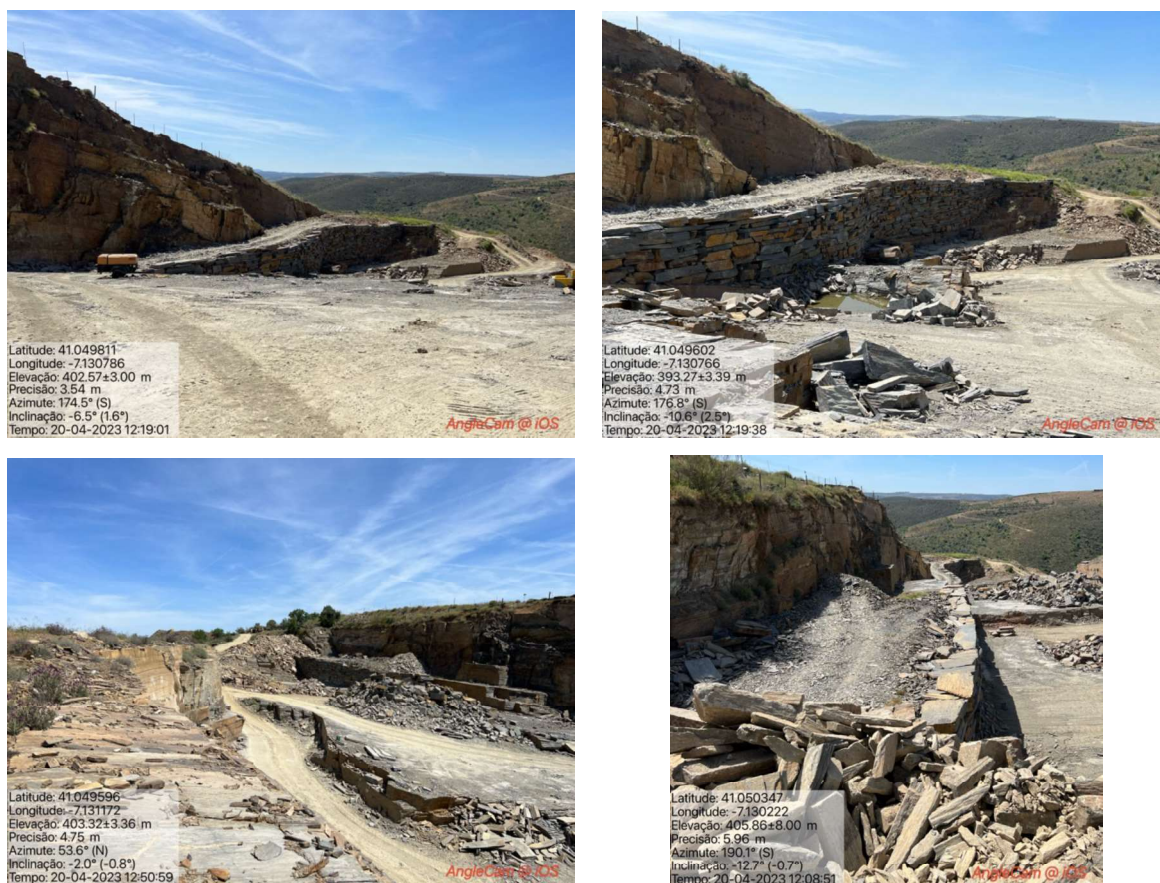
Figure 9: Photographs of the implemented landing showing the implementation of the smoothing and stabilization measure of the steeply sloping slopes with the creation of a raised landing at the base.
