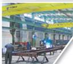
Calderaria Welding construction
