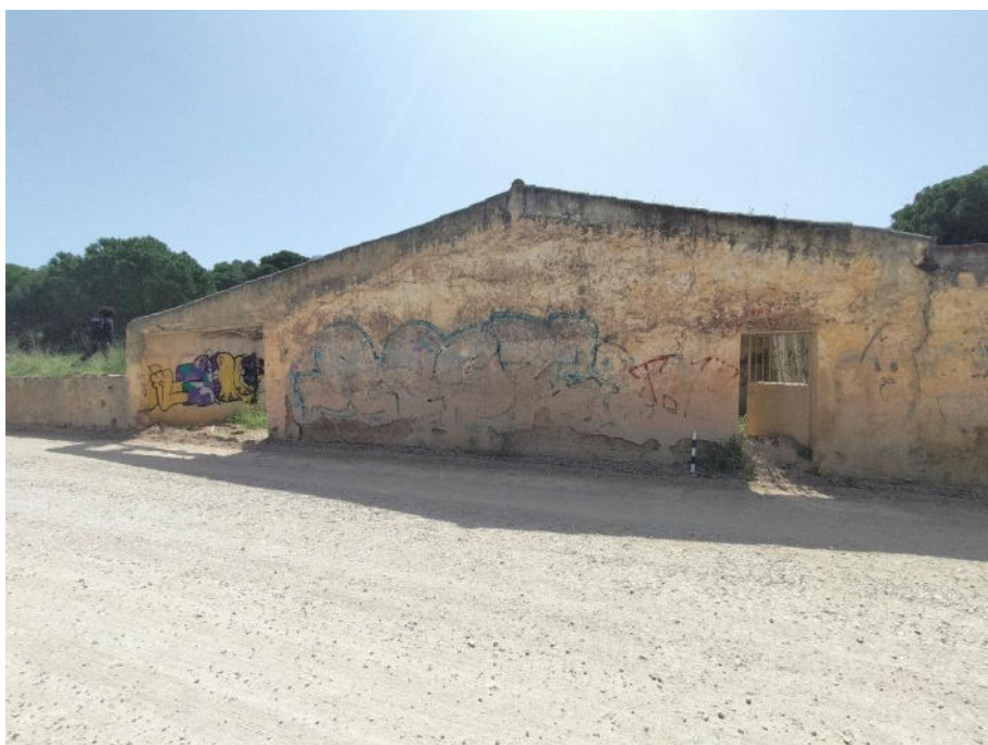
Figura 52. Fachada principal Alfamar 4.
