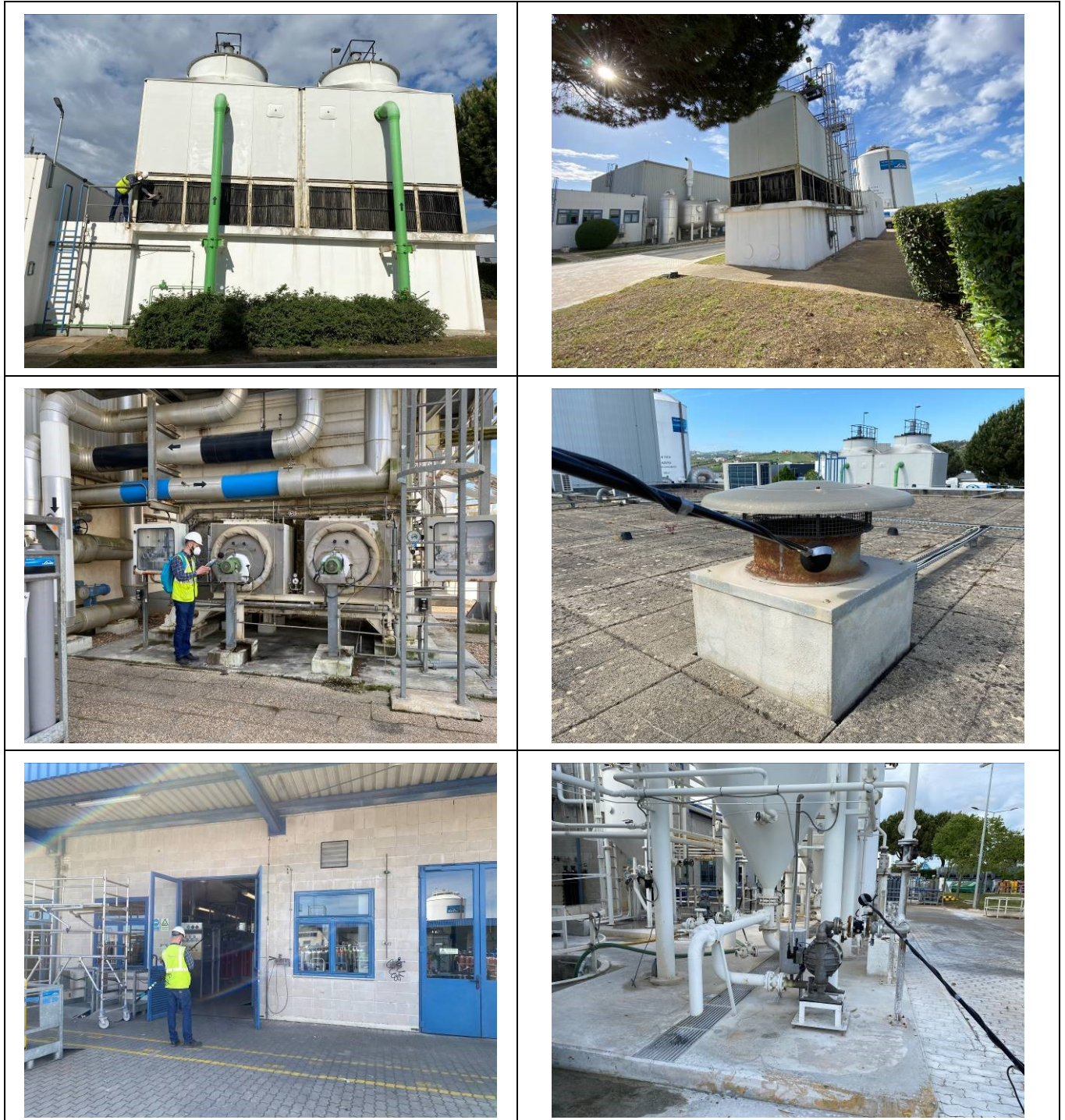
Figure 5-2 – Examples of close field sound measurements to characterize noise sources.
